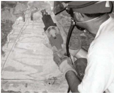
Figure 6 ▲ Cutting a wood panel
