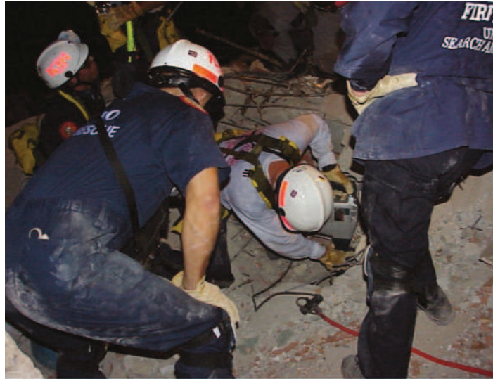
Figure 11 ► Breaching during a vertical approach
