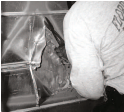
Figure 5 ▲ Cutting sheet metal
