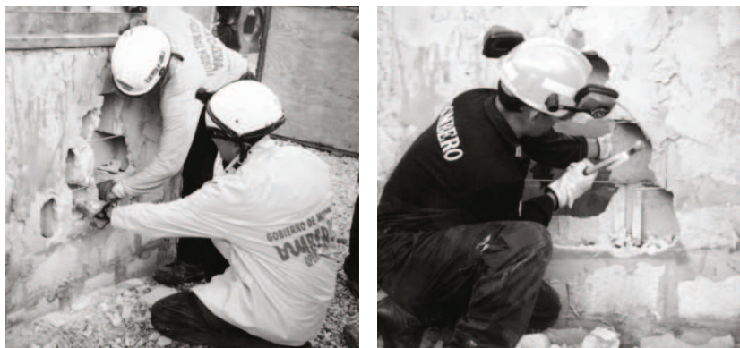
Figure 7 ► Breaching concrete block
