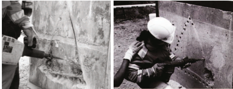
Figure 10 ► Breaching on horizontal approach
