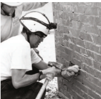
Figure 8 ▼ Breaching a brick wall
